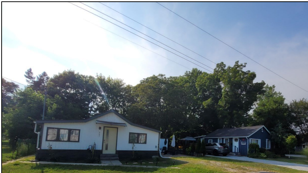
Photos 1 – North (Source: Pillon Abbs Inc.)
